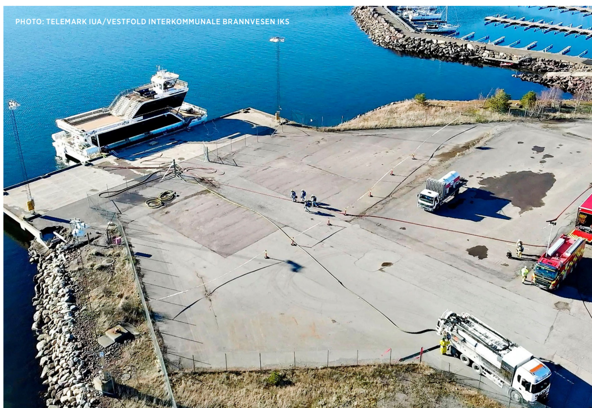
Four firemen on the way to the incident with VIB's self-developed connections to BRIM on day four. Nitrogen and extractor truck are ready, the operation to eliminate the explosion hazard is underway!
